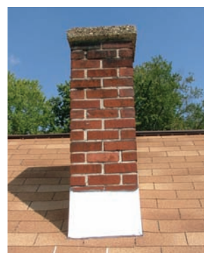
Disintegrating chimney
